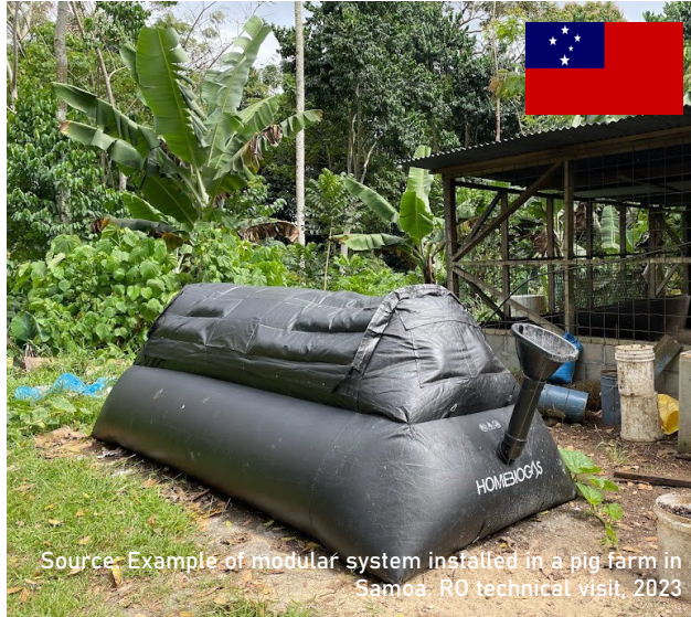
MNRE Modular Anaerobic Digestion Systems, Samoa Treatment Capacity: 540 TPY CAPEX: 41,500 USD Mitigation reduction potential: 9,000 tonCO 2 e
